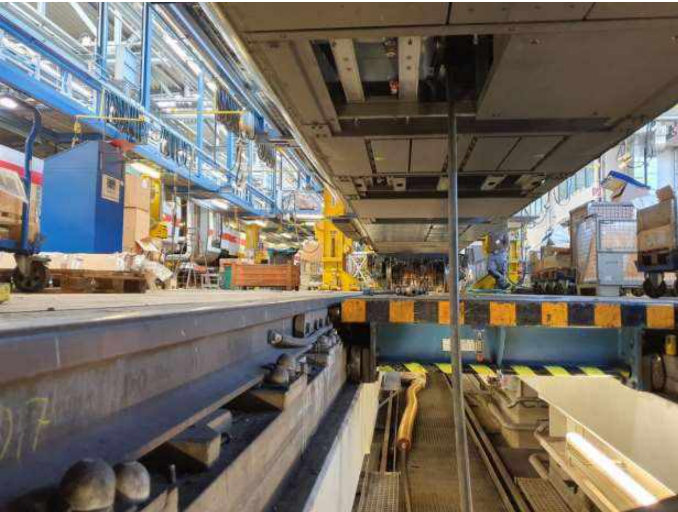
Manual cleaning of pneumatic pipes in the railway area using TubeMaster
