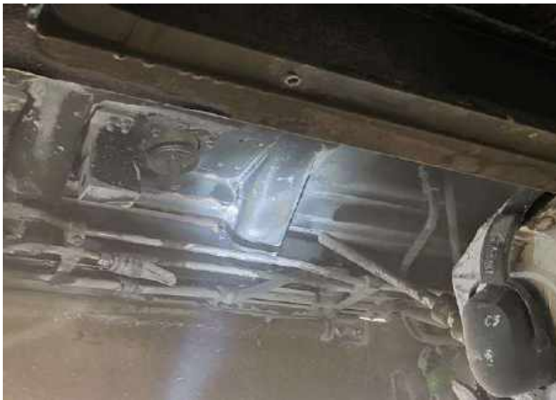
< Paint stripping for weld inspection
